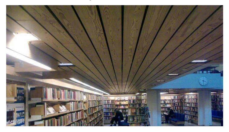
**HW02** offers protection to B-s1,d0, K210 and/or El60 for wood substrates. It is a water based clear intumescent varnish, tested also on previously painted surfaces.
