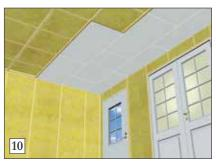
10) The rest of the rows of panels are installed in the same way, and the ceiling is finished.
