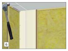
6) To prevent damage to the panel, a punch should be used when nailing to the final studding. Staples and screws can also be used on the panel.
