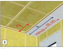
8) To find the length of the 1st panel in the 2nd row of panels, take the length of the 1st panel in the 1st row of panels minus 60 cm.
