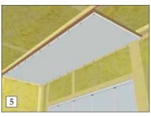
5) Install the 1st row of panels along string. Nail spacing is c/c 150 mm. NB: the panels to be installed 10mm from all walls.
